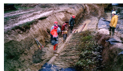
Work on embankments
